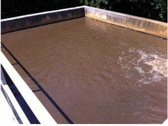
zones, denitrification is achieved within the flocs at a way higher rate than before where the DO concentration is not a limiting factor anymore like it is at the perimeter of the flocs. To reduce your TN in your effluent, we recommend you the following process to be executed:
