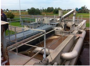
system has serious limitations due to the nature of the raw water: leachate mostly contains high amount of rotten organic substances, but also can have high heavy metal concentration, as well as high salinity. All above mentioned are serious inhibition factors for the biology, and can adversely affect treatment efficiency of the system.
