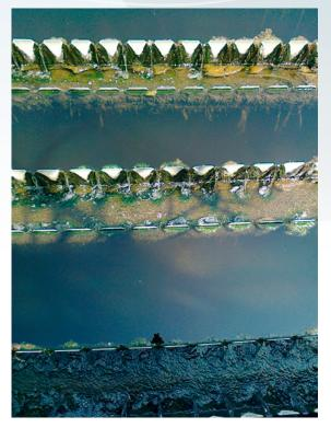
be adjusted. As a result, sludge washout from secondary clarifiers can be stopped or it will decline significantly. The effluent parameters of the overloaded plant can be optimised, moreover they may be brought down below the mandatory limits with trouble-free operation (COD, BOD, TSS, NH4-N, TN, TP). The process of nitrification in the activated sludge is usually hurt or stopped by overload. By Bioclean TM treatment the nitrifying ability of the overloaded plant can be totally restored.
