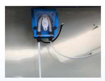
The unit is easy to operate without headache. Continuous dosage is done by a peristaltic pump. The net liquid volume of Malatech-C Dosing Unit is designed to be emptied by the peristaltic pump in 1-week time, so you need to refill the unit once a week. The delivery head of the pump is several meters, so the unit is not restricted to gravity, it can be placed way below the dosing point.
